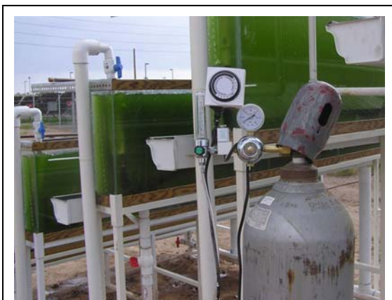
Figure 8. CO 2 supply system.
